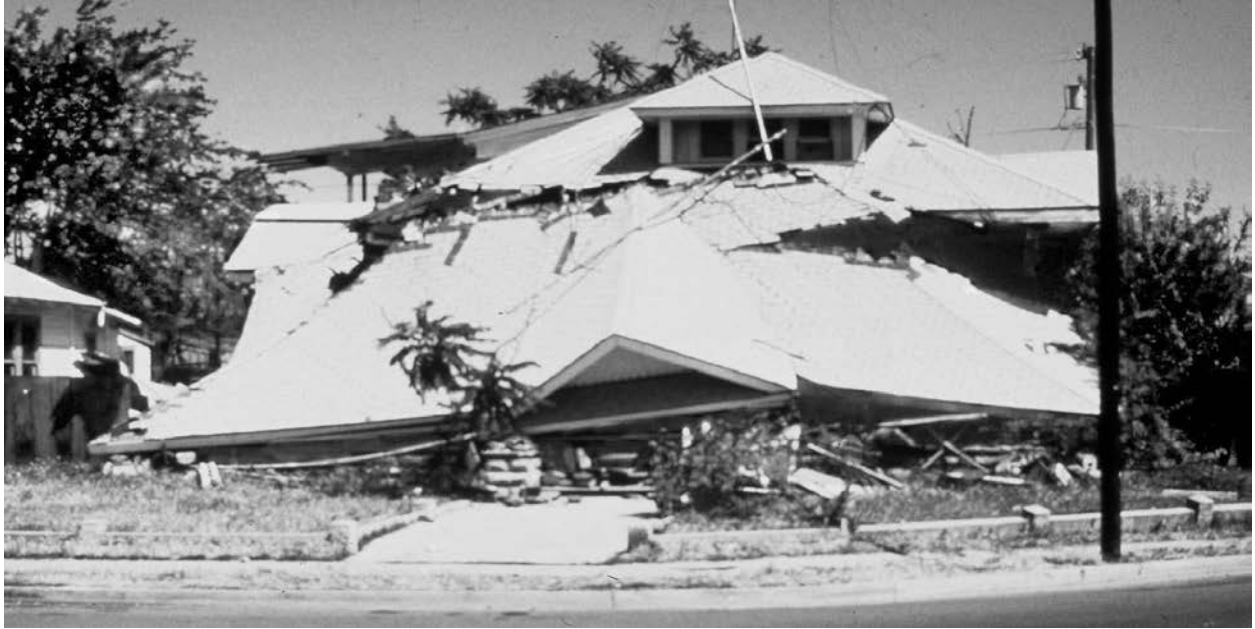
Photo 2 of 2: Numerous aftershocks occurred within the next few days, causing portions of the already-weakened structure to collapse.
