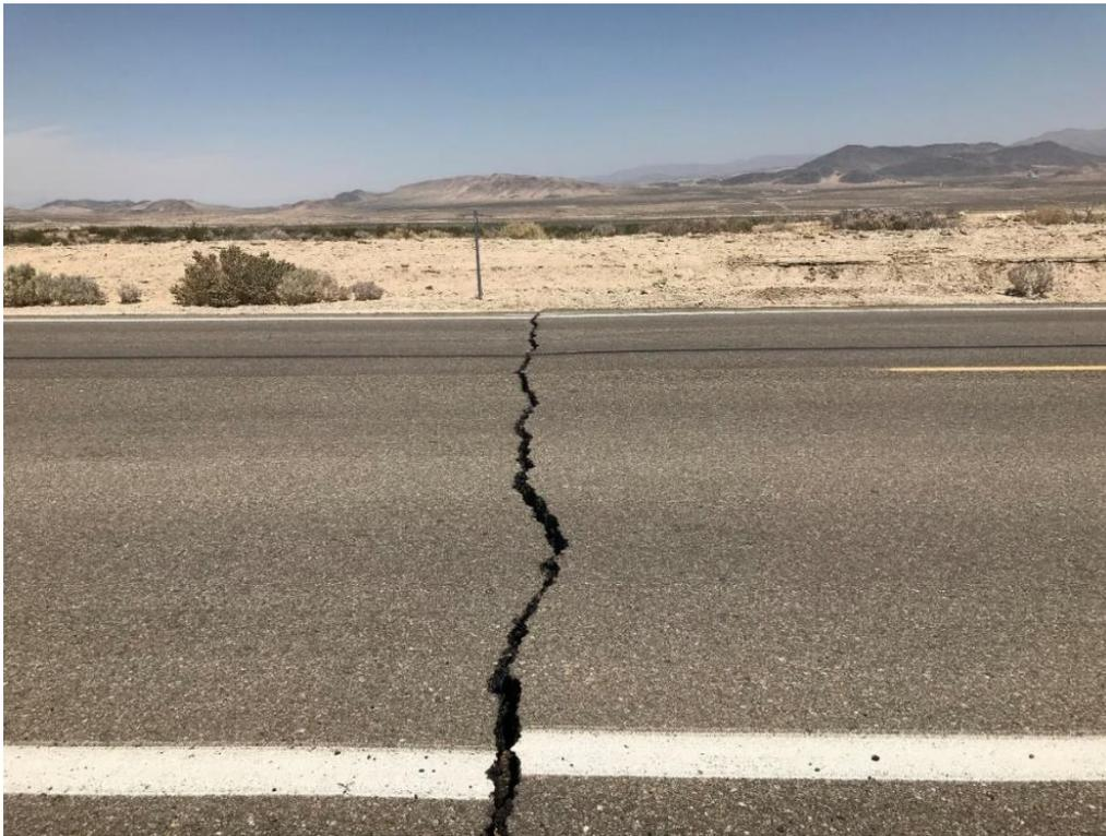
*Ground movement caused a crack and offset the painted lines on Highway 178 near Ridgecrest.*
